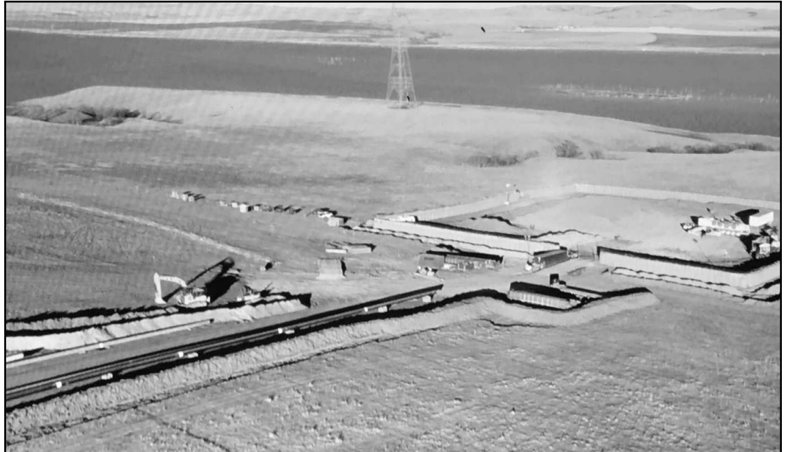
Aerial view of pipeline construction taken Nov. 3.
